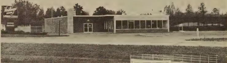
Our North Carolina Garden Shopping Center 4500 N. Independence Blvd., Charlotte
